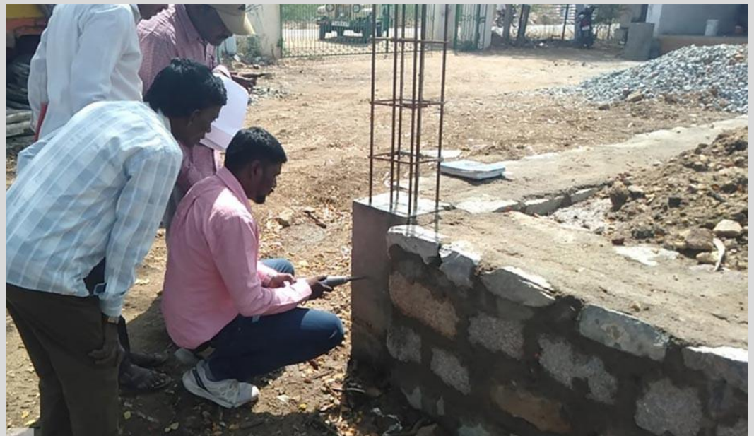
Rebound Hammer Test Conducted for Concrete Columns
