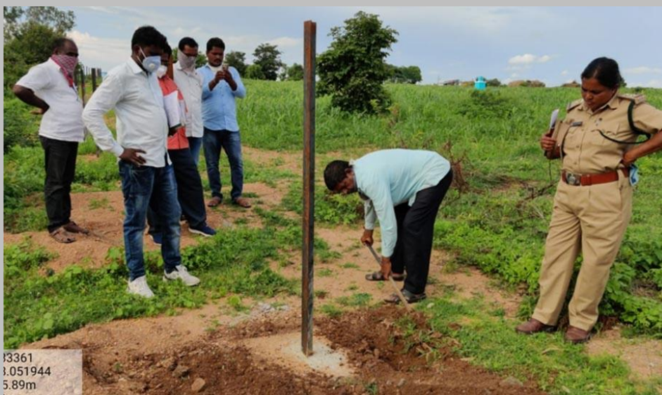
Checking the CC Foundation Sizes , during Post Construction of Work for Third Party Quality Control
