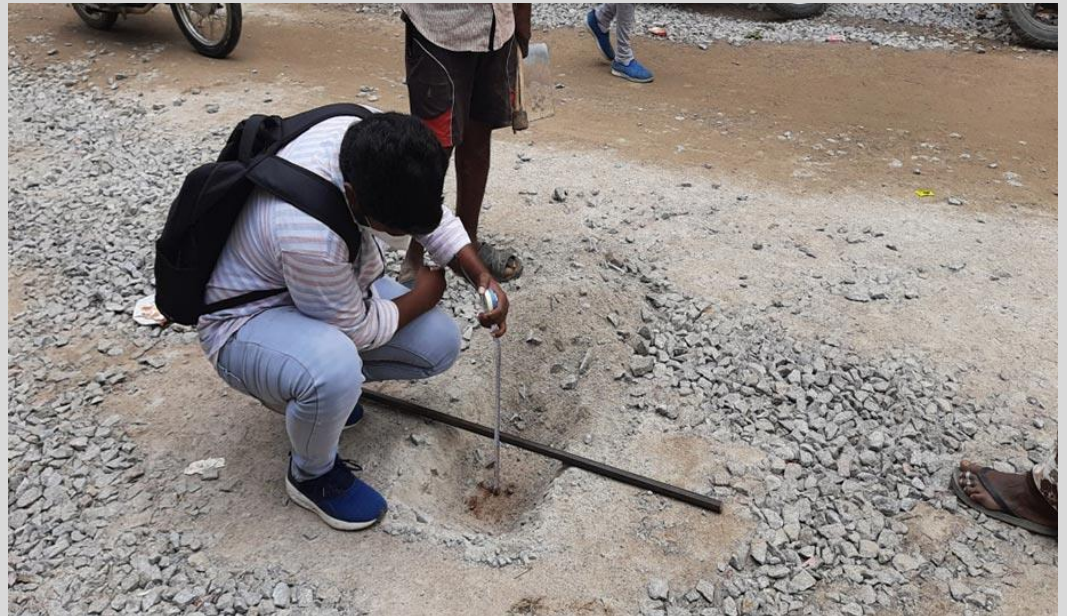
Checking the CC Foundation Sizes , during Post Construction of Work for Third Party Quality Control
